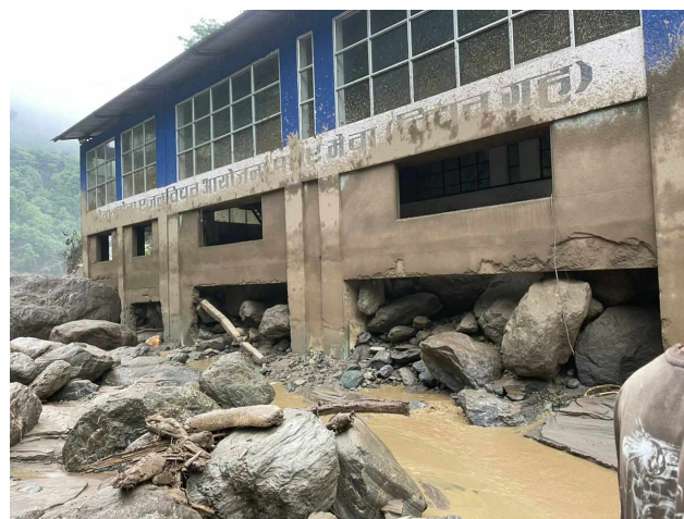
Figure 9. Damage to the Hewa HEP due to the flood on 16 June 2018 (source: The Annapurna Express newspaper, 26 June 2023).
