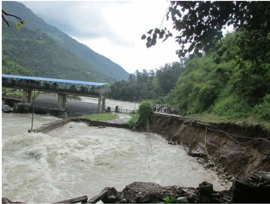
Figure 5. The Jure landslide damaged the road and headwork of the Sunkoshi hydropower project (source: Panthi, 2021).
