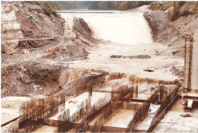
Figure 10. A diversion channel blocked at the Arun III Dam site due to a landslide (source: The Kathmandu Post newspaper, 1 May 2023).
