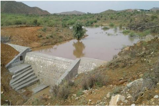
Figure 8. Closed type check dam.
