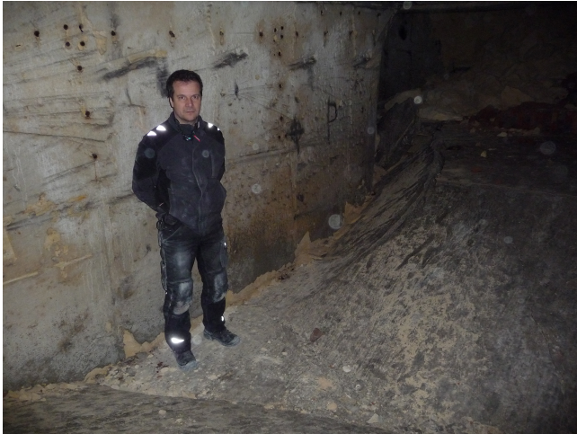
Figure 8. The strongly tilted mine floor in the collapse area of the Heidegroeve.
