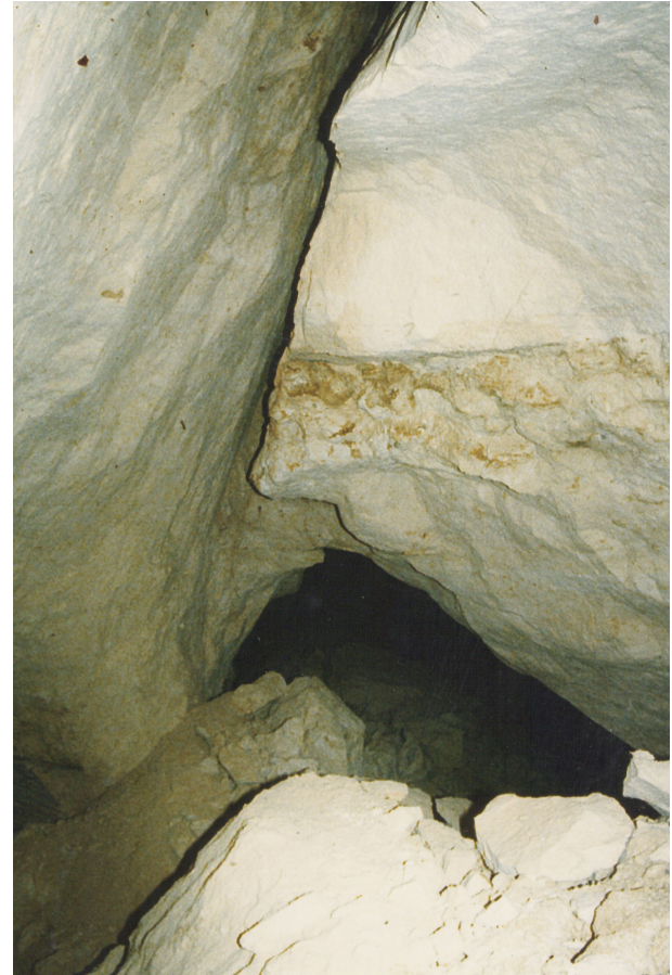
Figure 4. Collapse-induced fault in the rock overburden of the Heidegroeve.
