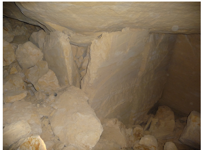
Figure 7. Collapsed pillar in the northeastern chamber of the lower mine system. The debris slope to the left gives access to this mine level.
