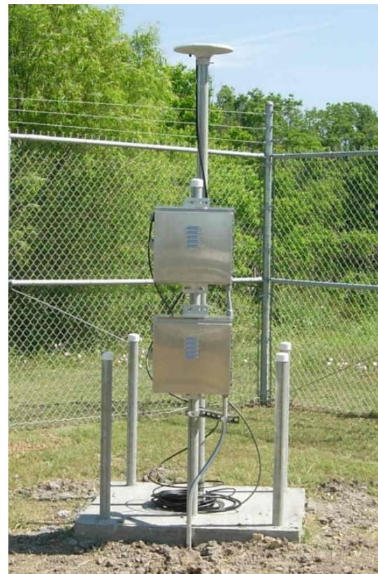
Figure 2. Subsidence monitoring station located near Texas City, TX, USA.
