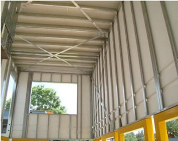
**Figure 1.** Interior view of the cold-formed steel structure.
